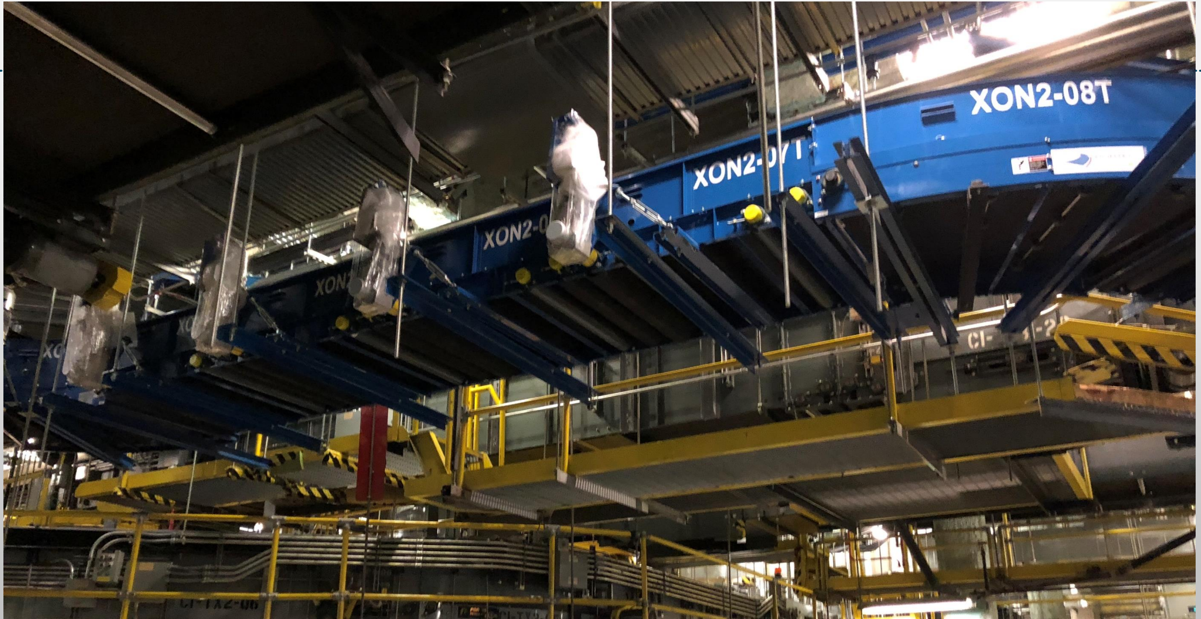
New Conveyor Installed
